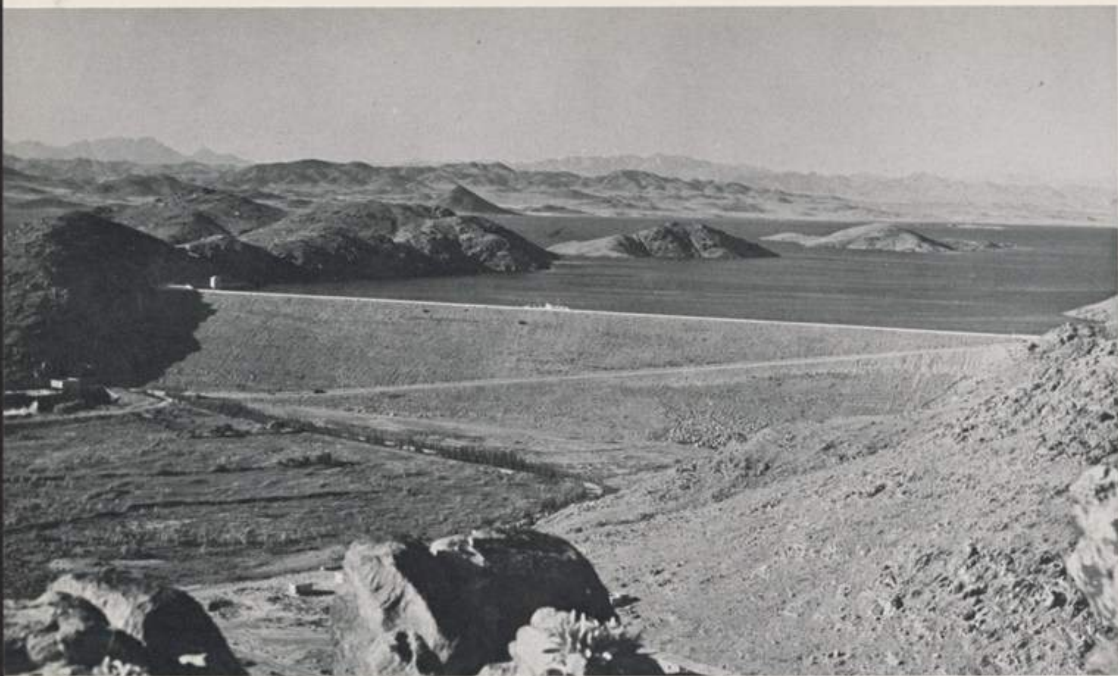
Kajakai and Arghandab storage dams will be tapped for power development.
